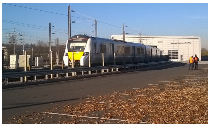
New Siemens' depot at Hornsey
